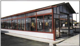
ning, and what Siegel called "an extremely involved process", the pair came up with a thermopane glass and polycarbonate building. The material is described as "indestructible plastic." The side walls are 11 feet high and made of glass, while a polycarbonate "knee wall" separates the glass from the ground. The roof is glass as well.
